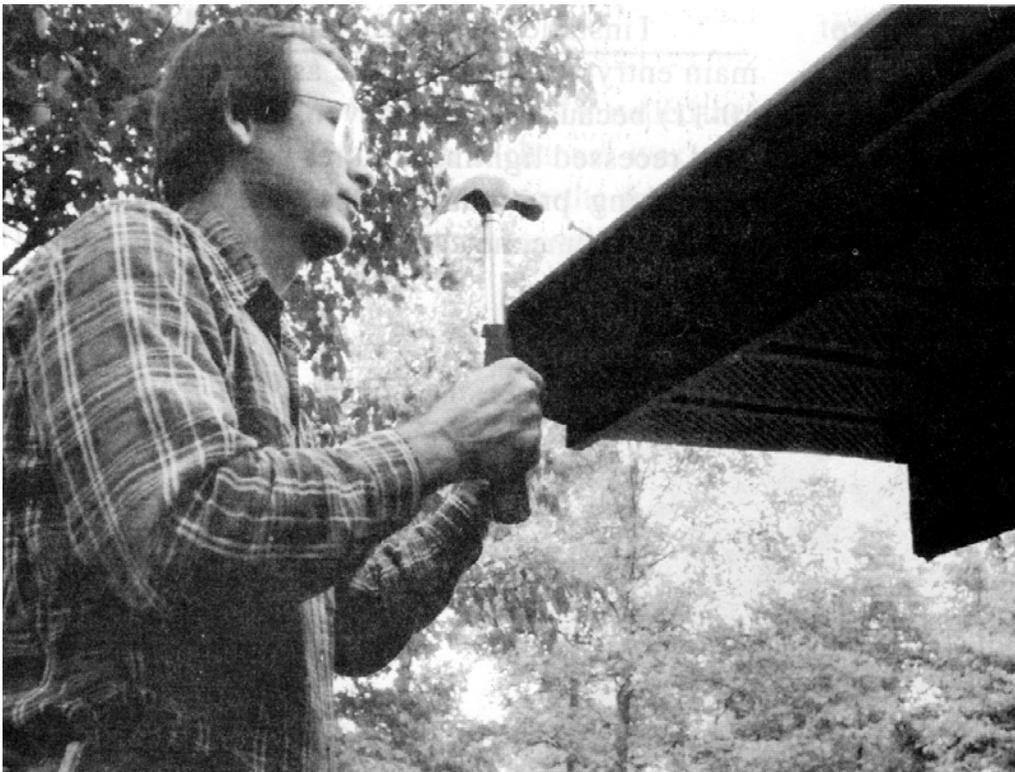
**Figure 10-12.** *Installing gutters.*
