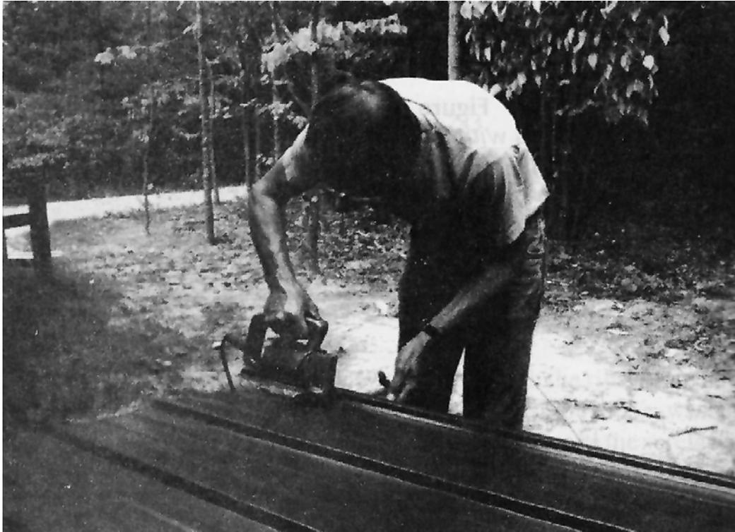
**Figure 7-6.** *Cutting sheet roofing with an electric shear.*
