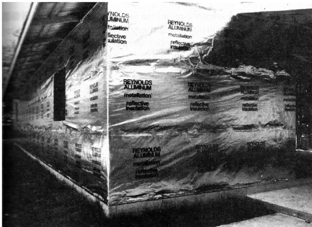
**Figure 8-4.** *Completed wind barrier.*
