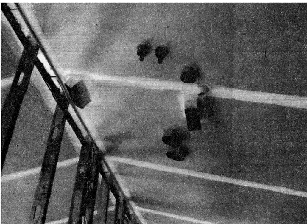
**Figure 13-9.** *Ductwork sealed to drywall.*
