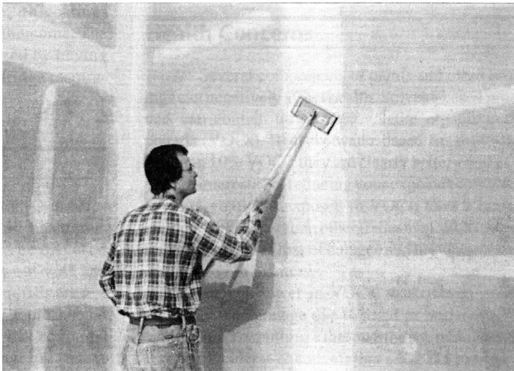
**Figure 20-7.** *Sanding the joint compound.*
