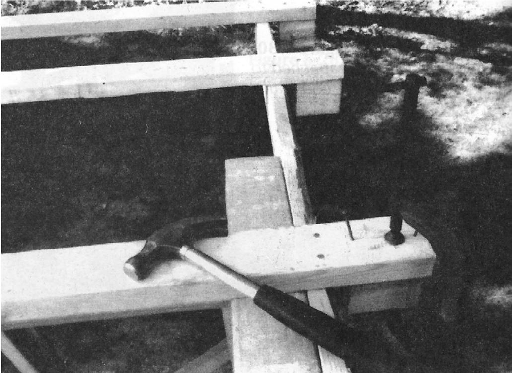
**Figure 6-32.** *Attaching blocking at purlin ends.*
