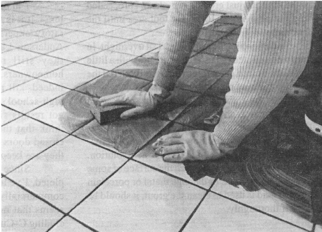
**Figure 22-8.** *Removing excess grout with a damp sponge.*
