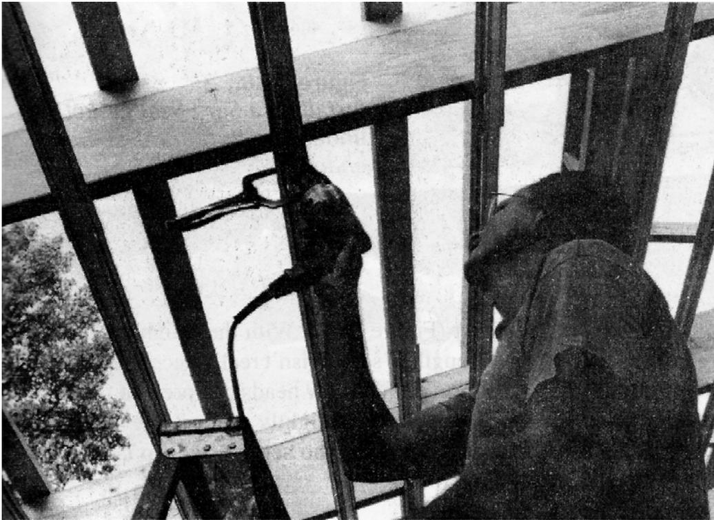
**Figure 6-34.** *Splicing two hat channels.*
