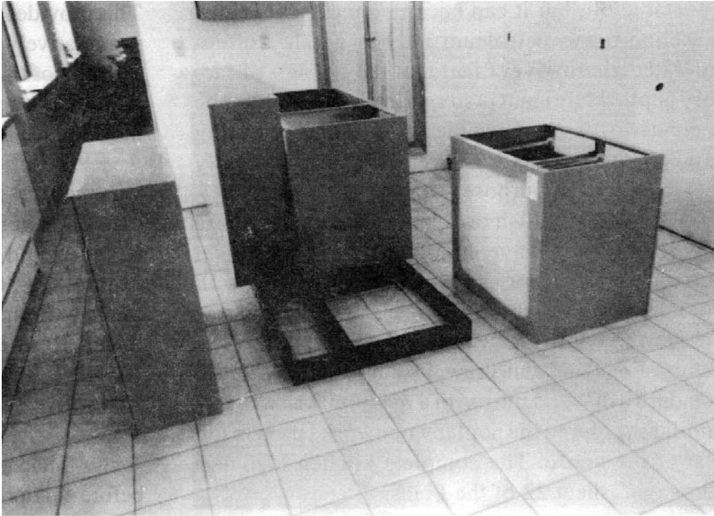
**Figure 23-4.** *Assembling base cabinets.*
