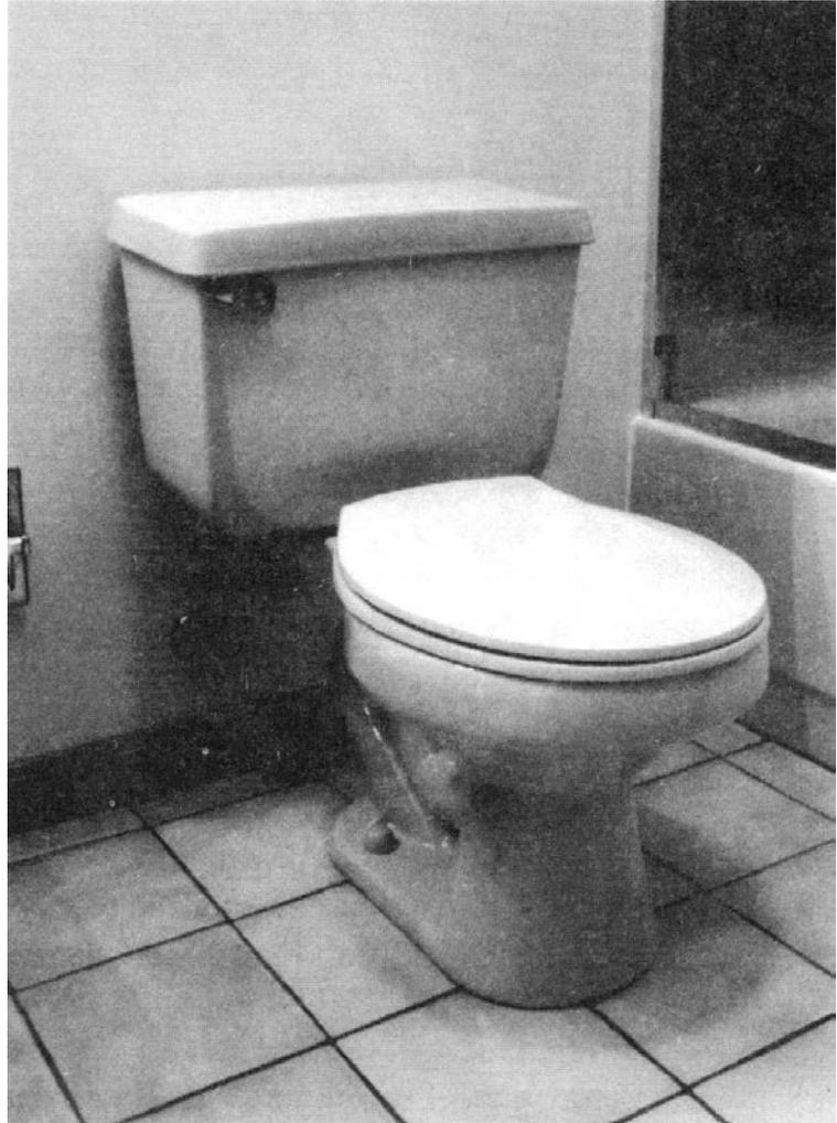
**Figure 24-3.** *Low-flow toilet with insulated tank.*
