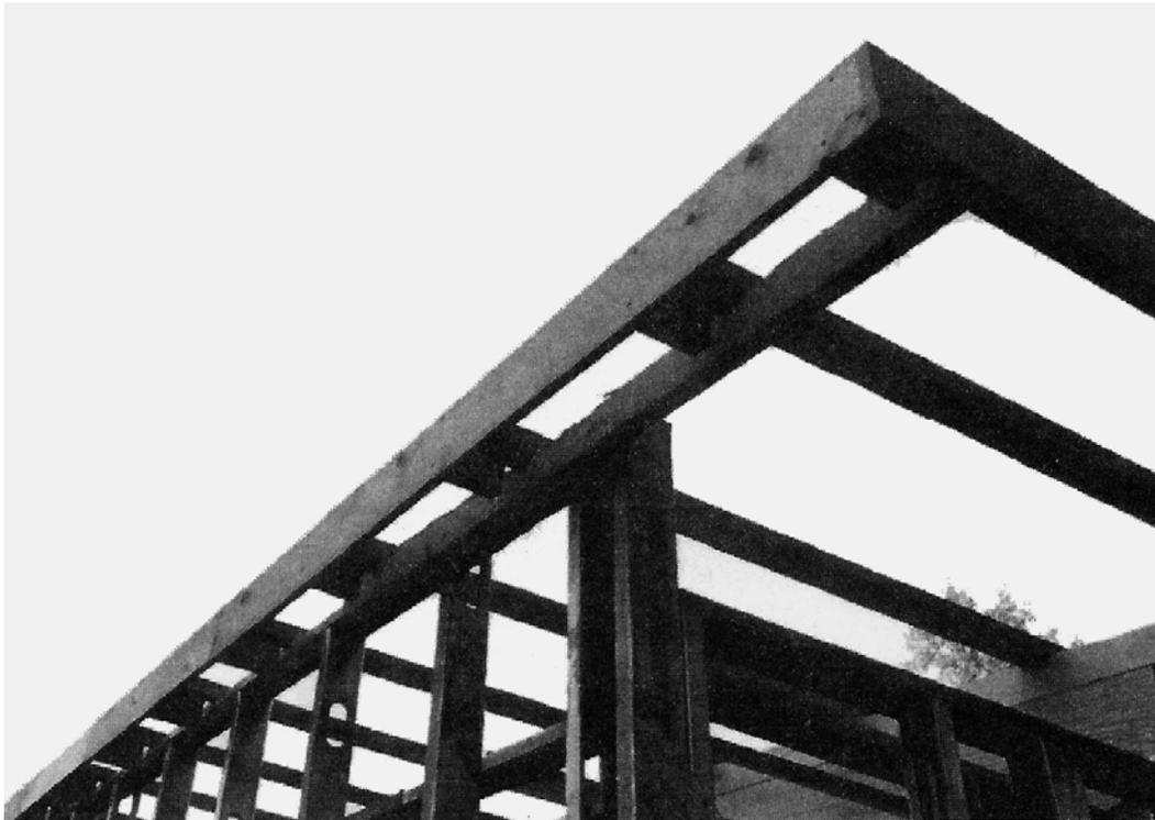
**Figure 6-30.** *2x4 outrigger rafters attached to end walls.*
