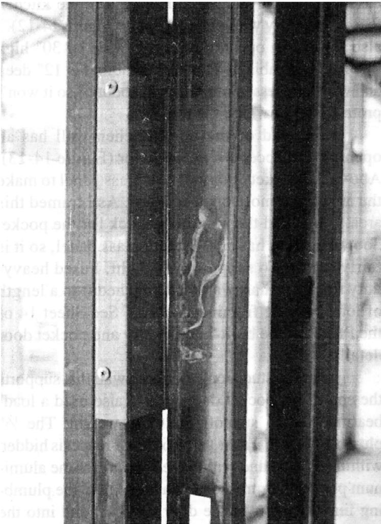
**Figure 14-18.** *“Blocking” for an electronic box.*
