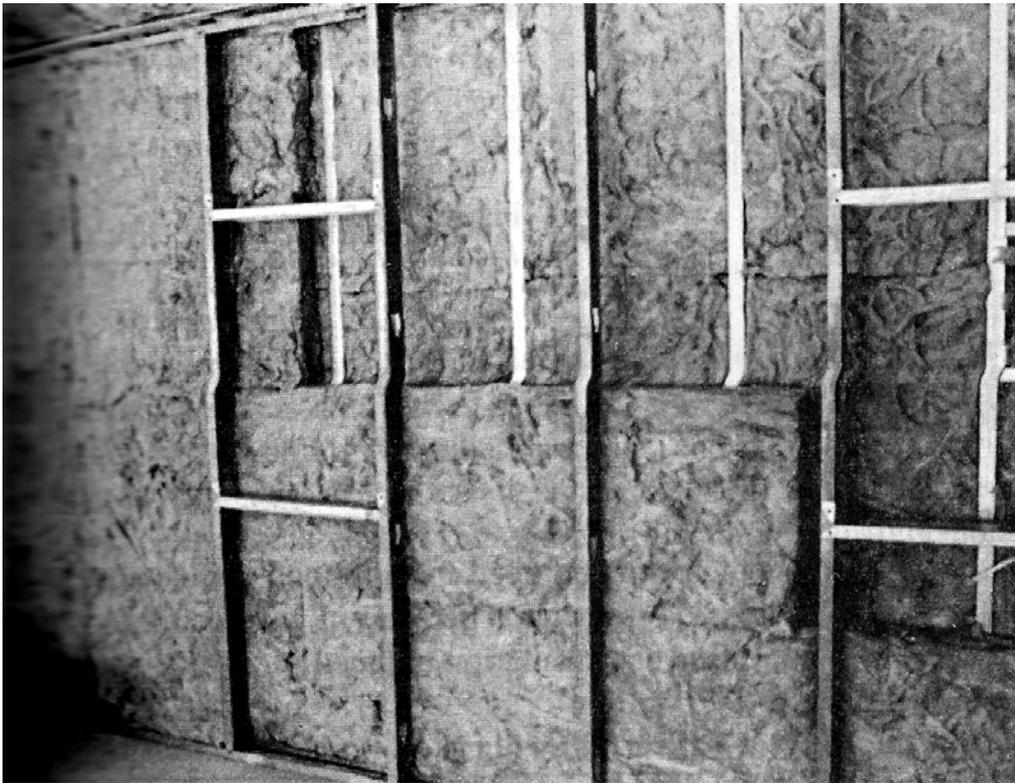
**Figure 12-3.** *Fiberglass and steel framing.*
