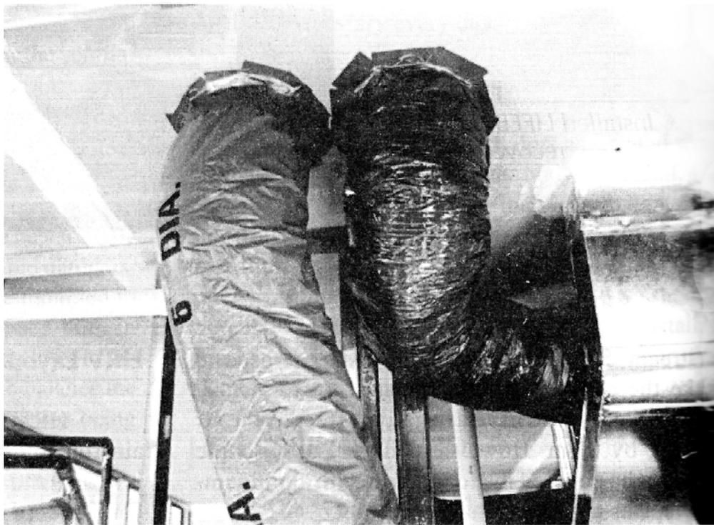
**Figure 15-13.** *Insulated ducts through the ceiling to the HRV.*
