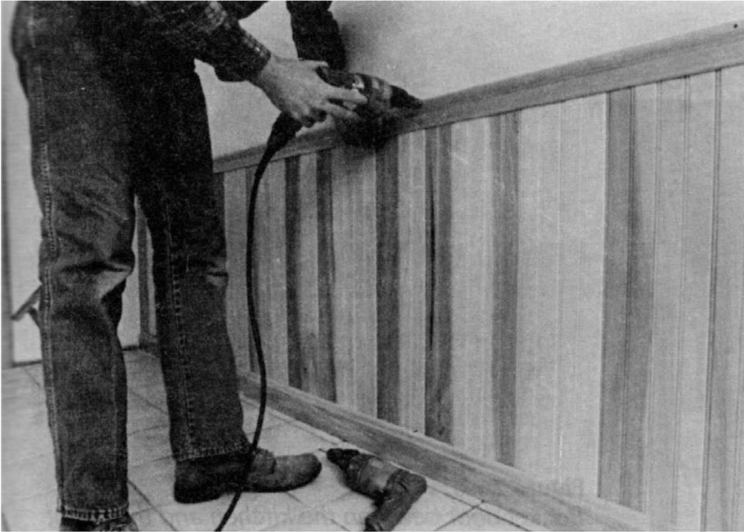
**Figure 26-6.** *Capping the wainscoting with a chair rail.*
