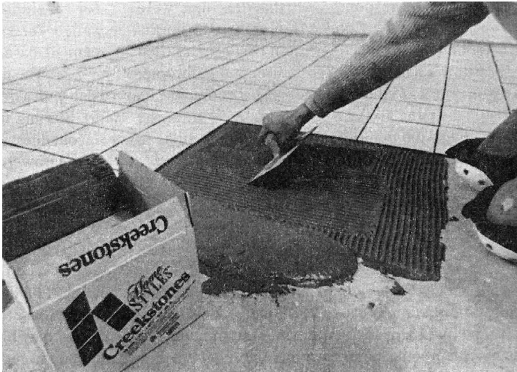
**Figure 22-5.** *Spreading the thin-set mortar.*
