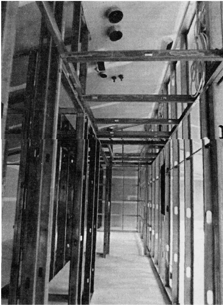
**Figure 14-11.** *Framing for hall ceiling.*
