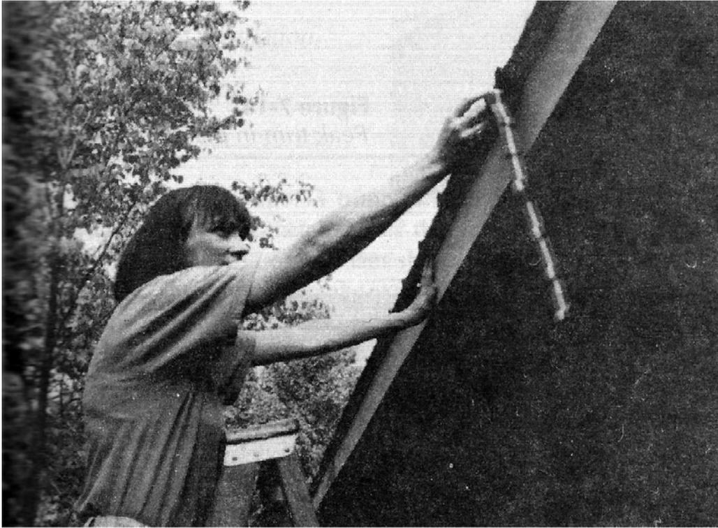
**Figure 7-13.** *Installing foam gaskets.*
