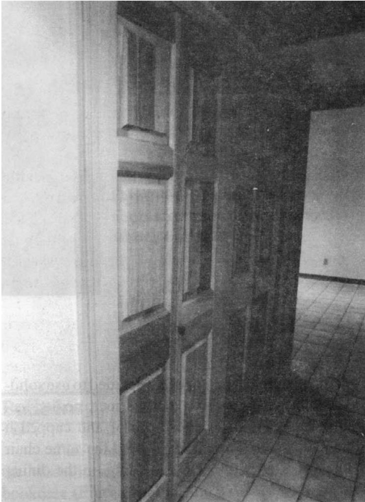
**Figure 26-2.** *Solid wood interior bi-fold doors.*
