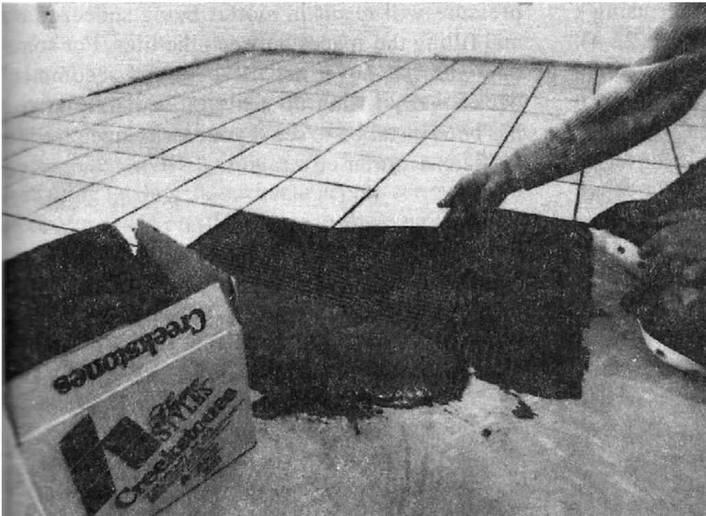
**Figure 22-6.** *Setting tile in the thin-set mortar.*
