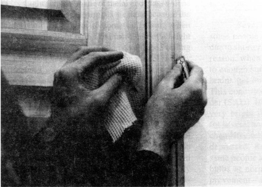
**Figure 26-13.** *Using a putty stick to fill over nail and screw heads.*
