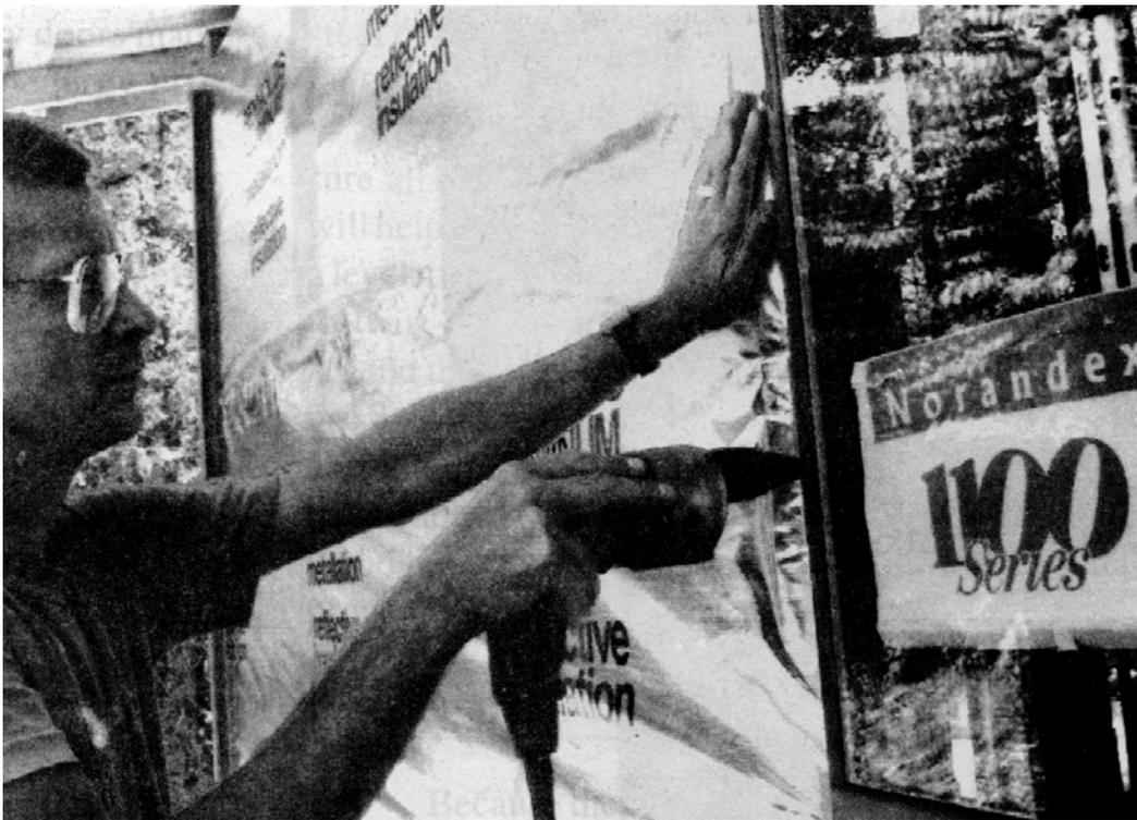
**Figure 9-2.** *Installing windows.*
