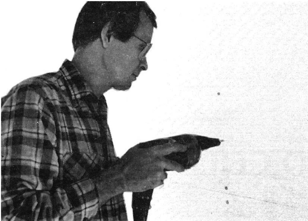
**Figure 20-1.** *Installing drywall screws*
