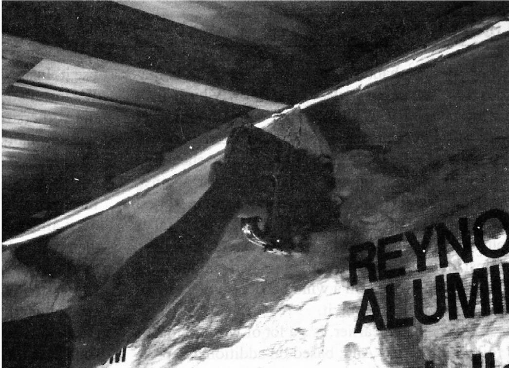
**Figure 8-3.** *Stapling the wind barrier to the rafter ends.*
