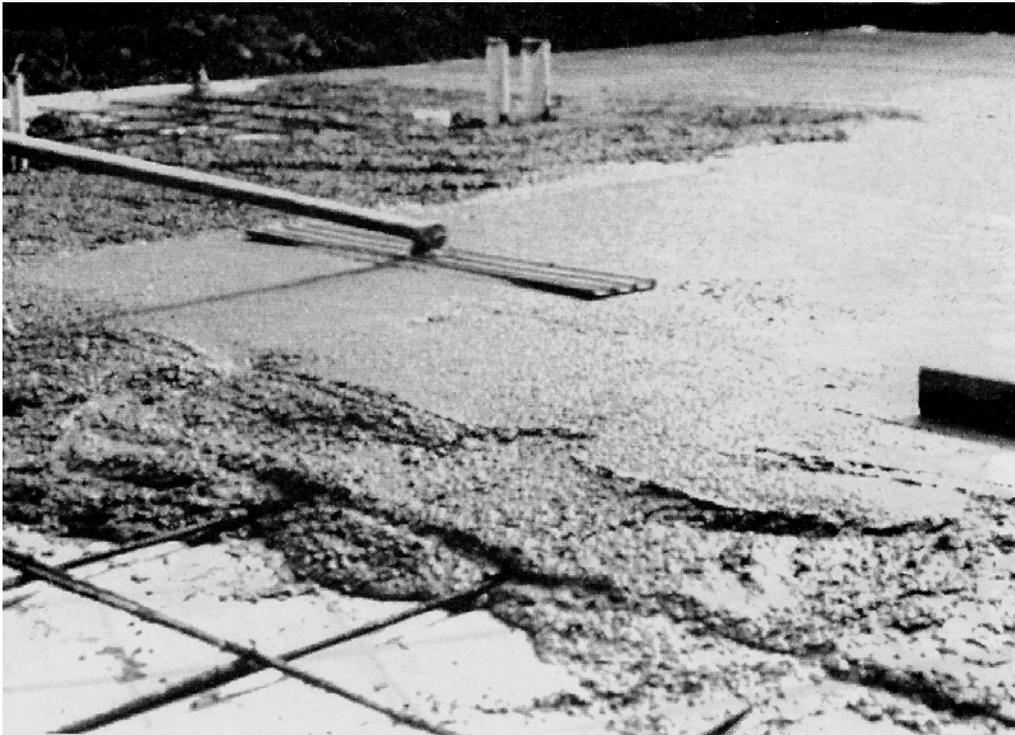
**Figure 5-17.** *Using a bull float to smooth the concrete floor slab.*
